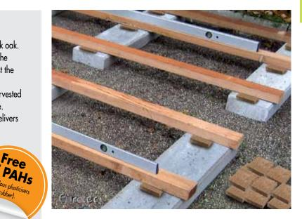
The cork pad spacers are laid between the deck substructure and the foundation/subsurface (self-adhesive on one side) and thus form a gap that aids constructive timber protection. The cork pad spacers are available in three sizes. These are 3 mm, 6 mm and 10 mm thickness/height (see Fig.). In addition to the advantages already mentioned, useful side effects of using the spacer include the option to adjust the height of the substructure and that the loads are distributed evenly.
