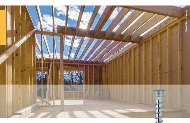
The KonstruX ST is a universal fully threaded screw for connecting timber frame elements such as posts and cross-beams. Measuring 6 mm in diameter, the KonstruX ST ZK is especially suitable for connecting slim timber frame elements grouped in service classes 1 and 2.
